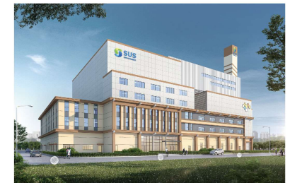
Makassar Waste-to-Energy Plant in Indonesia
