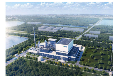
Nonthaburi Waste-to-Energy Plant in Thailand
