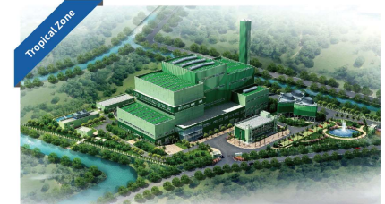
Sri Lanka Colombo Waste-to-Energy Plant
