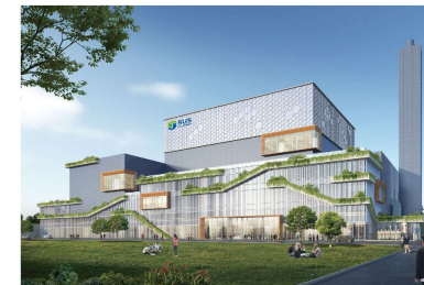
Ho Chi Minh City Tam Sinh Nghia Waste-to-Energy Plant in Vietnam
